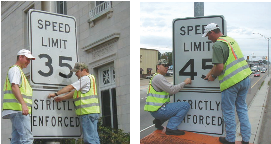
Figure 1. Installing updated regulatory speed limit signs
